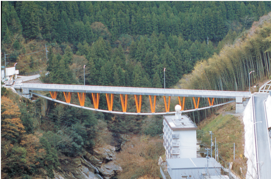
Rys.17. Most ukończony [8] Fig.17. Completed bridge [8]
