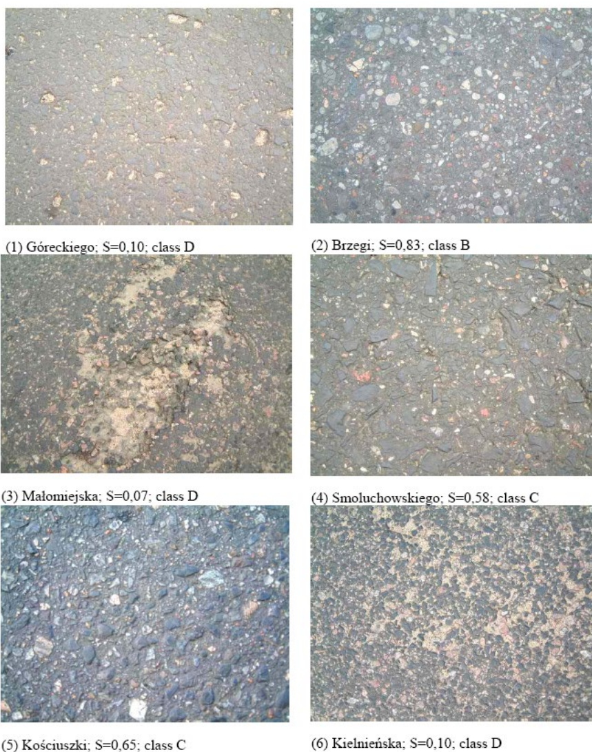
Figure 1. Pavements of tested streets in Gdansk and Gdynia, condition rating given under each photo, part 1
