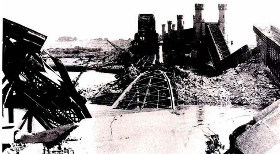
Fig. 3. War damages of bridges in 1938
