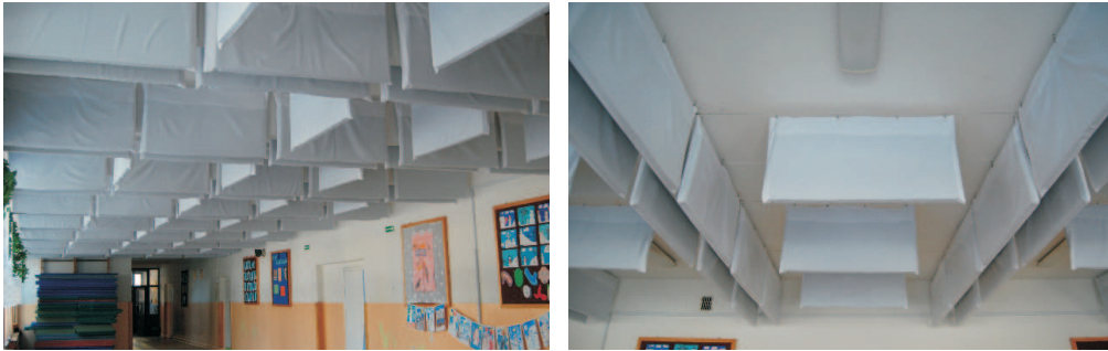
Fig. 1. School 1 corridor after acoustic adaptation.
