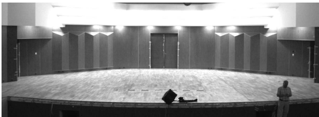
Fig. 6. Sound diffusing elements on back wall of the stage.
