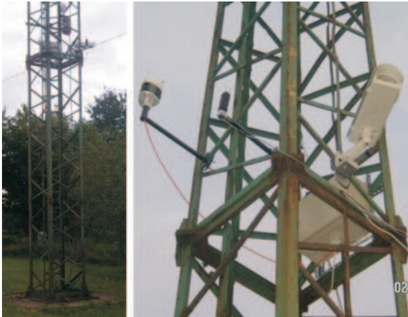
Fig. 10. Noise station installed for long term measurements in location 'C'.
