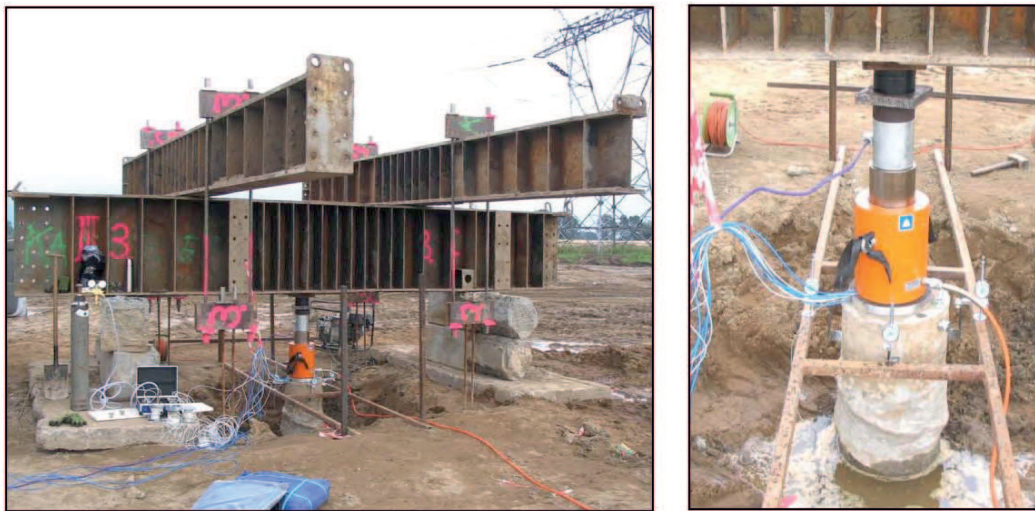
Fig. 7. Screw pile at static load test.
