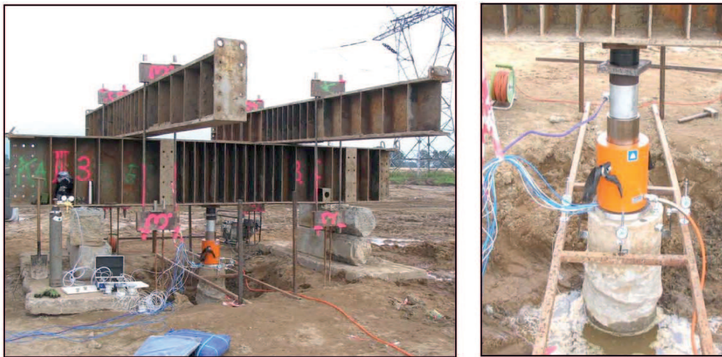
Fig. 7. Screw pile at static load test.
