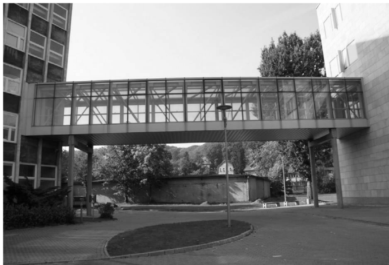
Fig. 9. View of measured foot-bridge.
