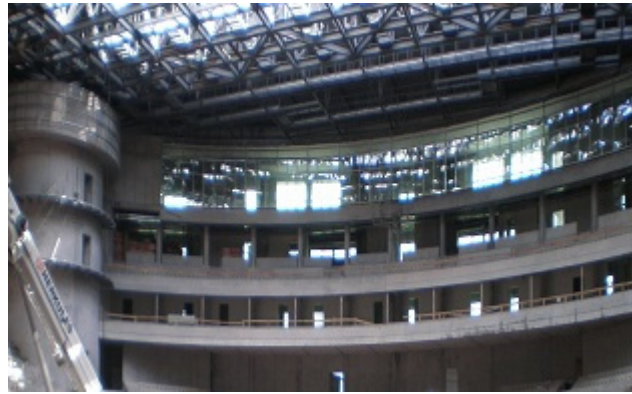
Fig. 3. View of the pylon and the girder of Hall.
