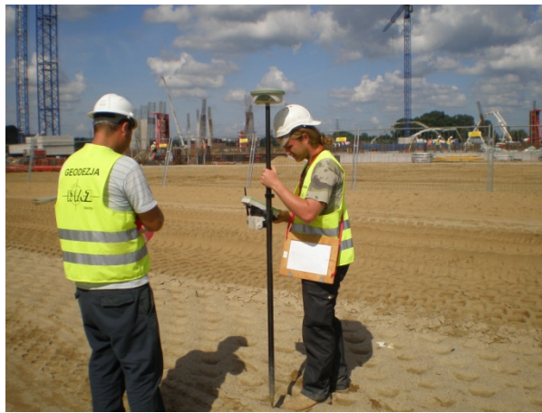
Fig. 8. Staking out axis of heads of reinforcing subsoil piles by means of GPS.
