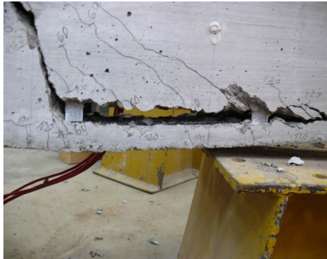
Fig. 9. Apparent sliding separation of the neighbouring stirrups from the main reinforcement in beam 1.
