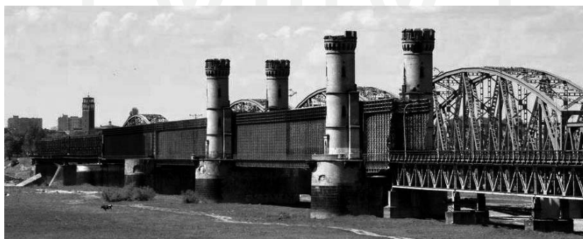
Fig. 2. A view of the current condition of the bridge
