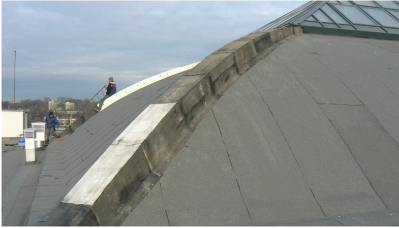
Fig. 18. View of the insulated ribs of the dome of Gdynia Seaport Dome (December 2013)
