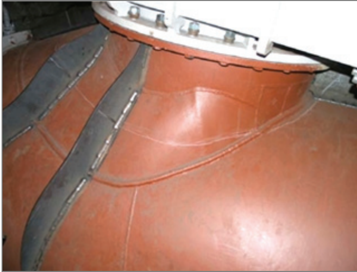
Fig. 18. Assembly of webs to the inlet pipe and the pipeline coating. Source: prepared by the authors
