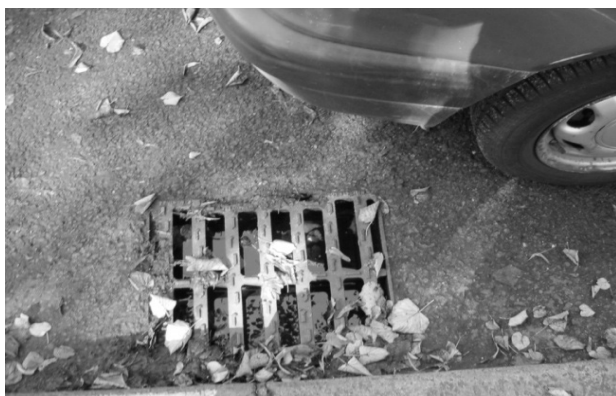
Fig. 1. Fallen withered Oak leaves blocking rain water discharge cesspits found at the side of roads (taken by researcher Nov. 2012).
