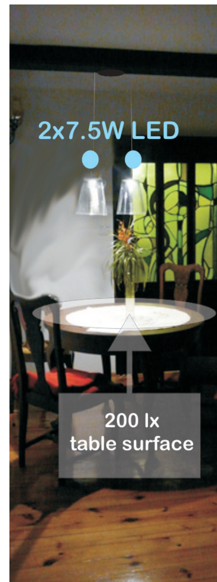
The new lighting for the writing task showing lux levels
