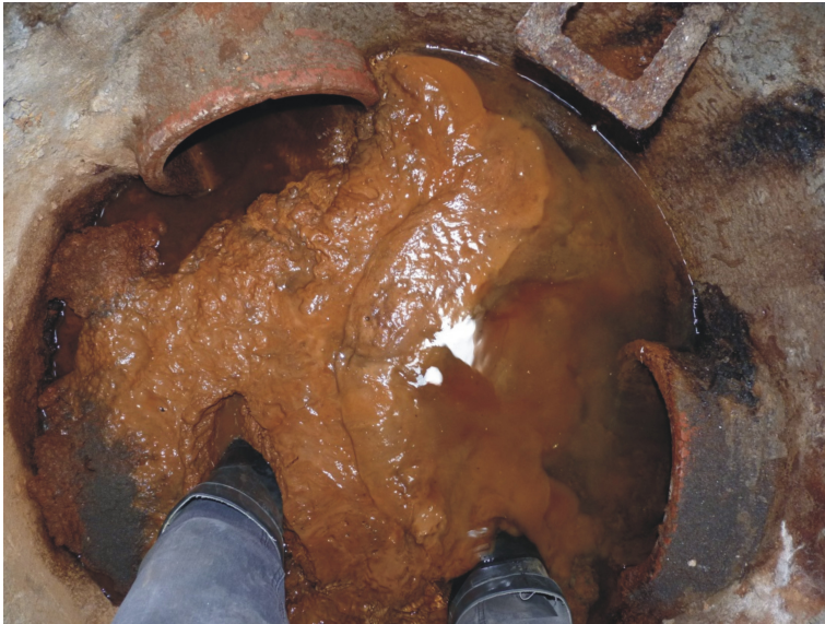
Fig. 3. Ferruginous substance in a well
