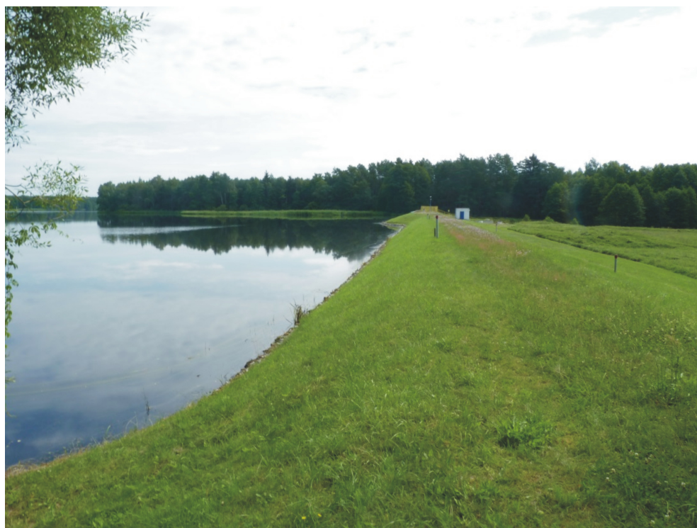
Fig. 2. General view of the Podgaje earth dam
