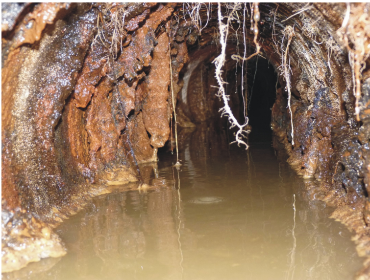
Fig. 4. Ferruginous substance in a pipe
