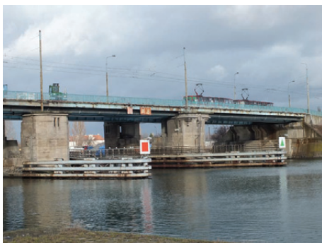
Fig. 1. Siennicki Bridge in Gdansk
