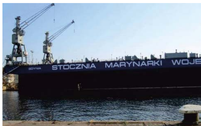
Fig. 10. Naval Shipyard Co floating dock of 135 m in length, and 35 m in breadth
