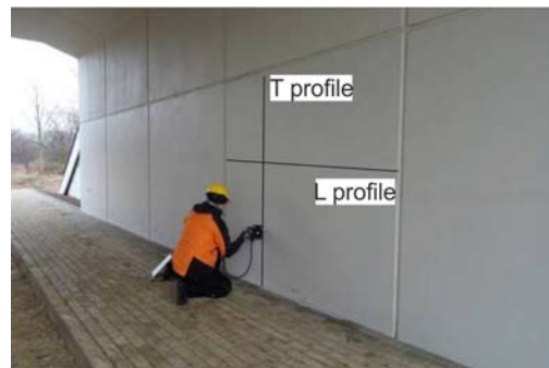
Fig. 8. Abutment of railway viaduct
