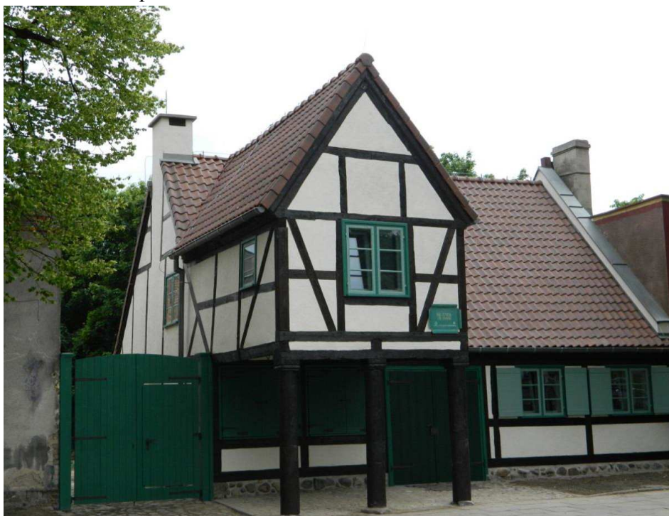
Fig. 1. Forge building after completion of construction-conservation work
