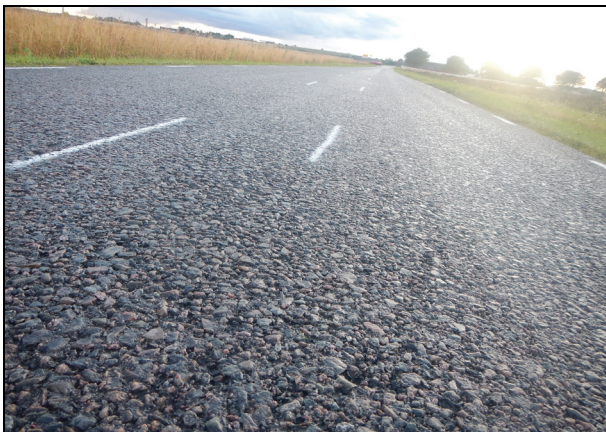
Fig. 7 View on test site in Rokinge (wet conditions).
