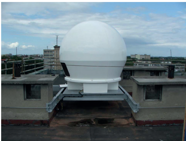
Fig. 1a. 1.5 metre HRPT-MetOp antenna in radome
