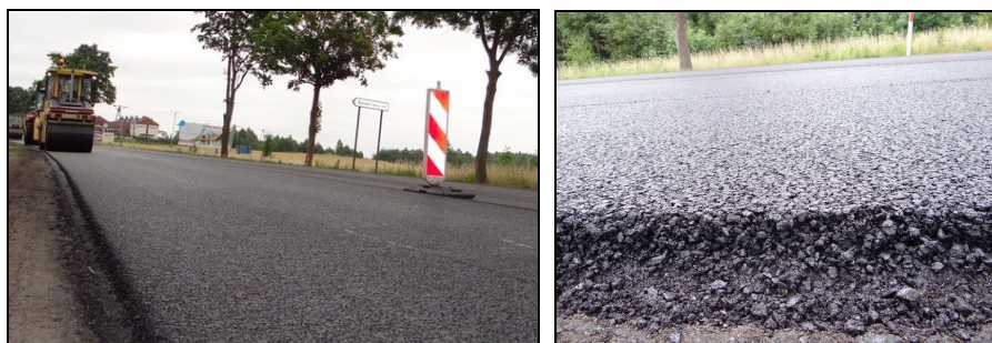
Figure 3. Building of the test SMA 11 section with polymer-rubber modified bitumen in wearing course
