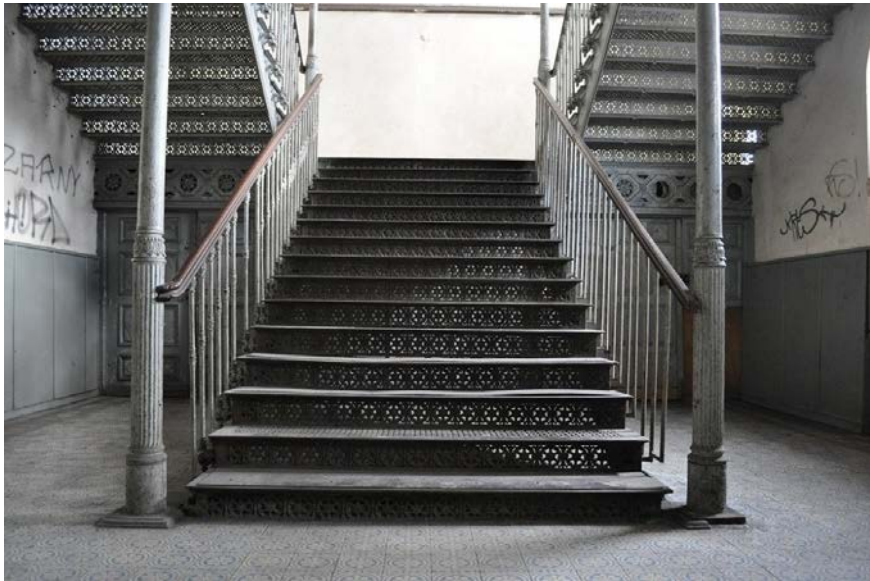
Fig. 1. Cast iron staircase: general view.
