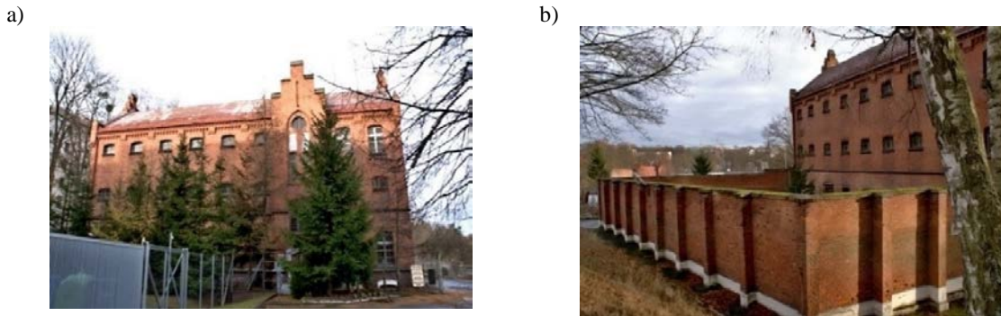
Fig. 1. Building of the garrison arrest: (a) from the south, (b) from the north with the perimeter wall encircling the prison yard.
