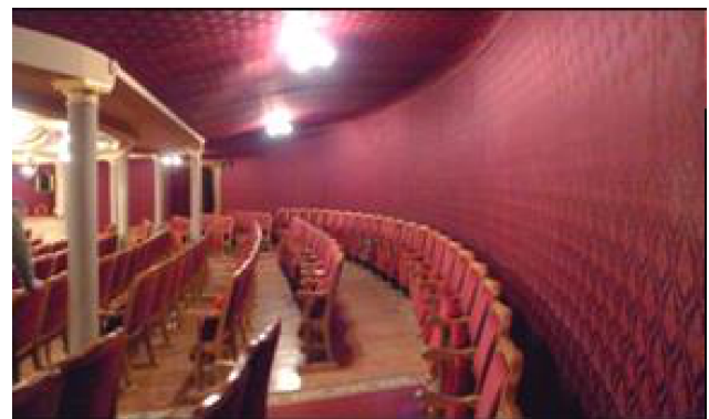
Fig. 8. The underbalcony space in the Lviv Opera House hall prior to installing the sound diffusing structures. The walls and ceiling were covered with a textile tapestry.
