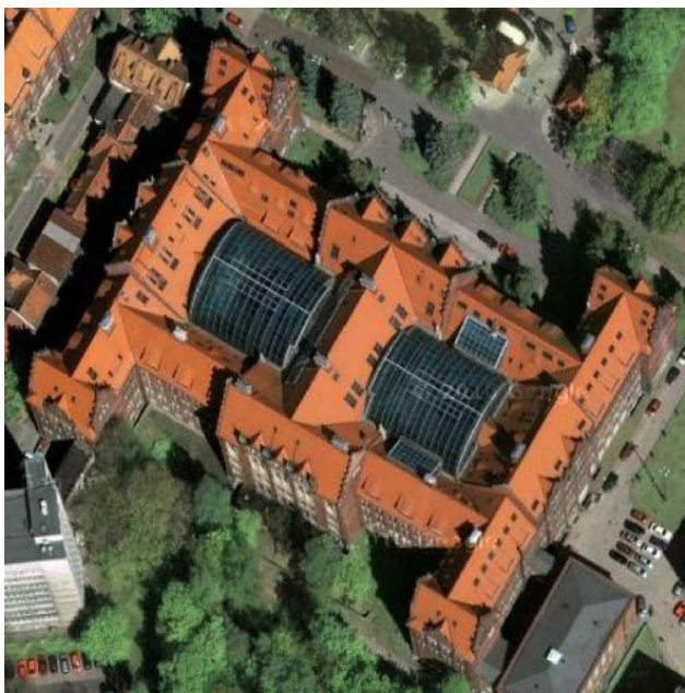
Fig. 18. Glazing roofs over Gdańsk University of Technology's main building courtyards (Google maps, 2015).
