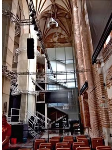
Fig. 4. The renovated St. John's Church in Gdansk as an example of combining sacral and cultural functions.
