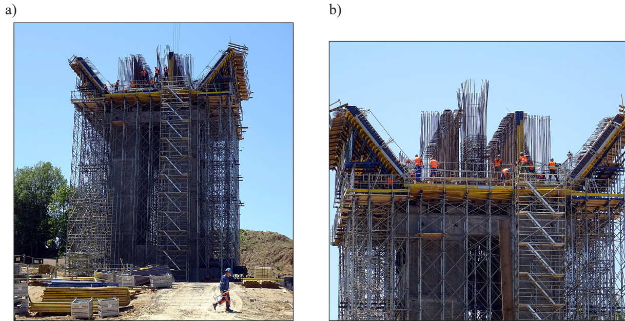
Fig. 4. First section on stationary scaffold (a), view of the deck section (b)
