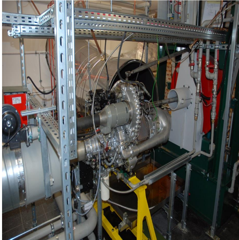
Img 1. View of a two-shaft gas turbine
