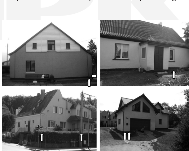
Fig. 1. Buildings tested for traffic-induced vibrations (arrows indicate the locations of vibration sensors)
