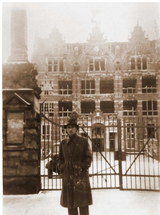
Fig. 2. View of the Main Building of the Gdansk University of Technology just after Gdansk was liberated, in March 1945 [www.pg.gda.pl]
