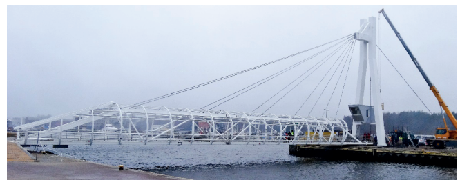
Fig. 1. Rotating footbridge for pedestrians over the Ustka port channel (configuration W1a)
