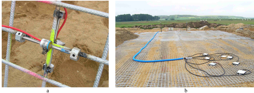
Fig. 6. a. Strain gages on the steel grid; b. Location of the protected sensors before backfilling
