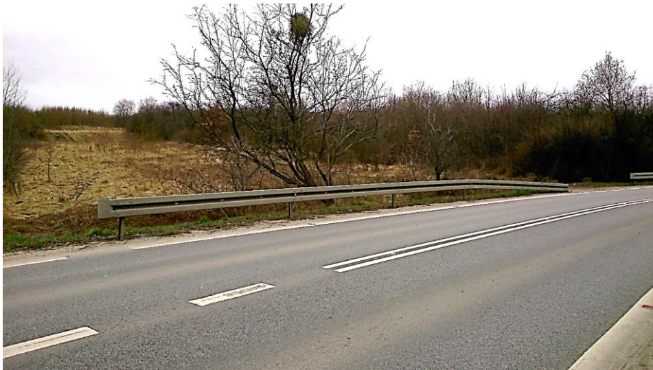
Fig.1: Short barrier erected at the roadside. Probably the tree is an obstacle to be protected.
