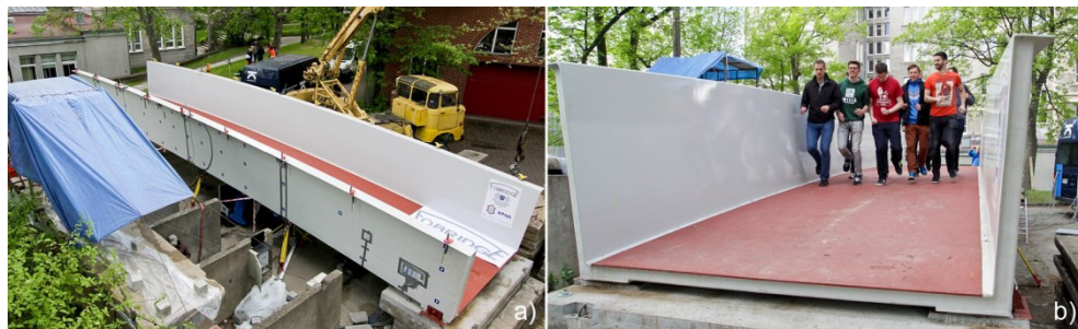
Fig. 8. GFRP footbridge constructed within Fobridge project.
