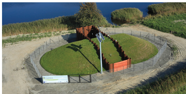
Fig. 2. The ready-to-use test stand – aerial view
