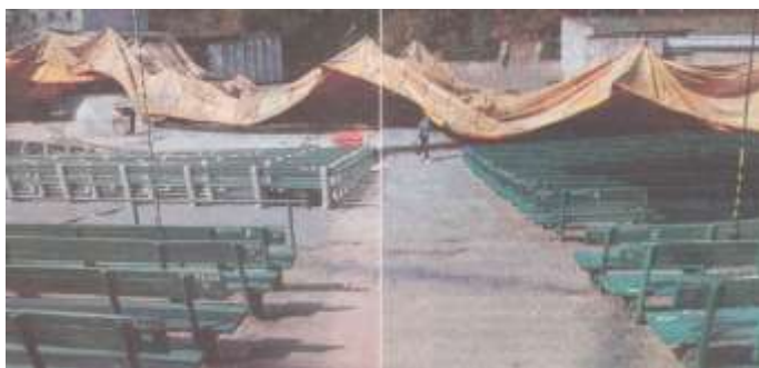
Figure 1. Putting down the roofing structure of the Forest Opera in Sopot (Poland) before winter season (Dziennik Bałtycki 2007).
