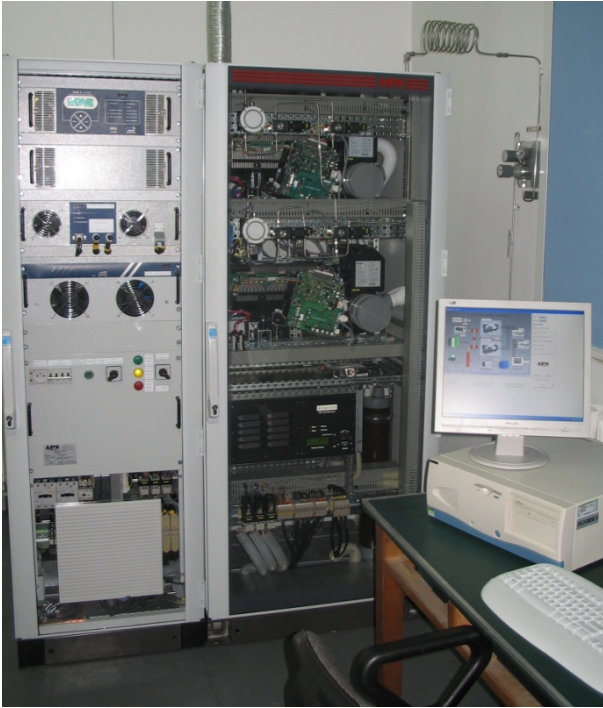
Figure 2: View of the module
