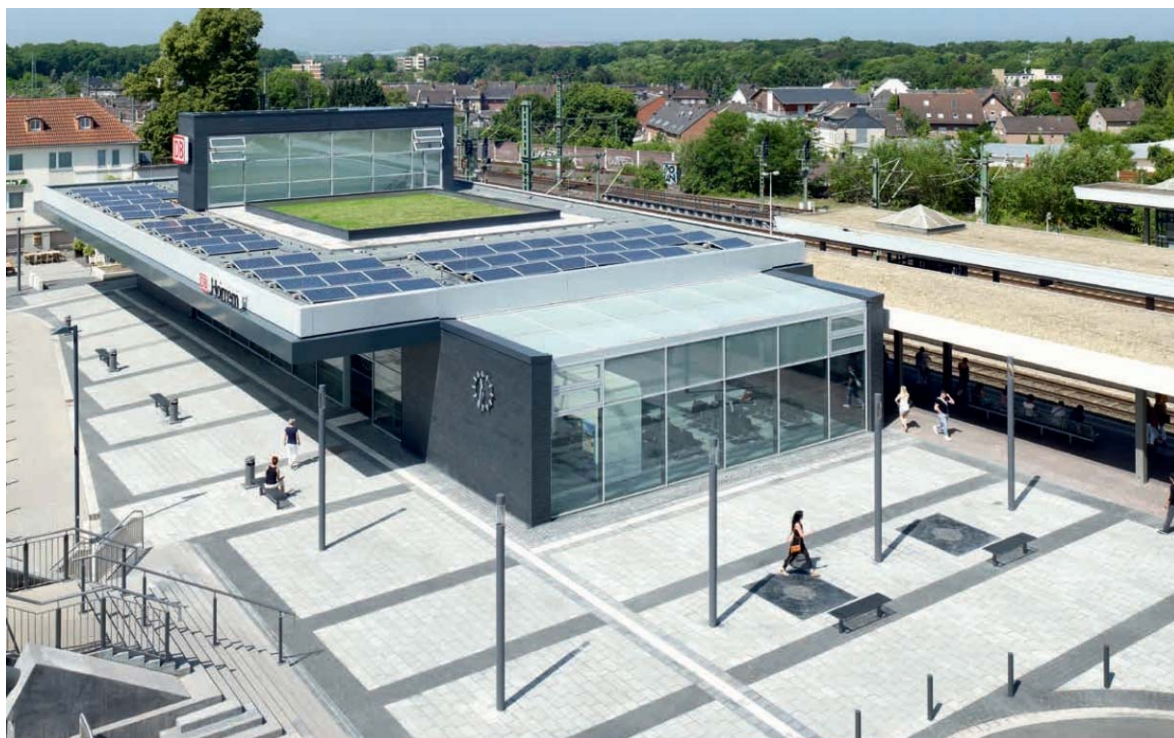
Figure 4. Green Station Kerpen-Horrem (DB Station&Service AG from [11]). Green roof and a photovoltaic system has been situated on the roof to cater the demand of energy and heating at the station
