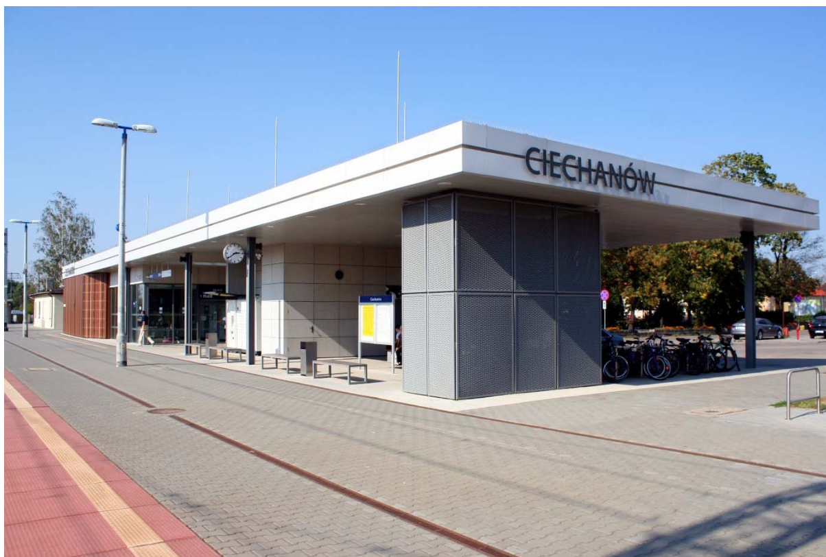
Figure 5. Innovative Railway Station in Ciechanów (D.Zański). A seasonal waiting room shaded and well protected from the rain by a large field of the extended roof. Also a place for bicycle racks, vending machines, storage lockers and ATMs
