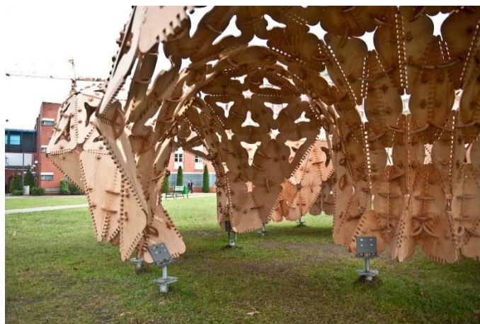
Figure 6. Pavillon was made of plywood panels [38]
