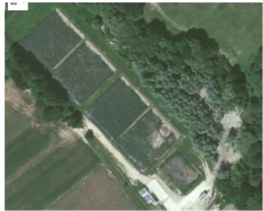
Figure 1. Scheme of technology of the analyzed wastewater treatment plant with the application of Kickuth-type wetland and Google view.
