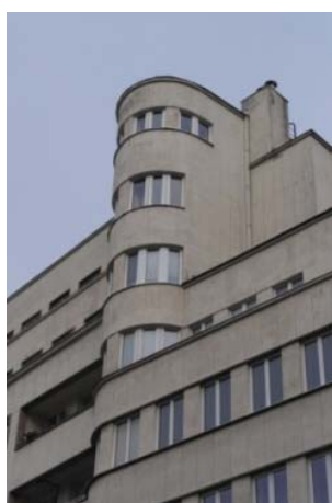
Figure 4. BGK residential complex, Gdynia, 3-ego Maja street, Poland
