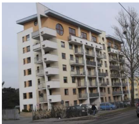
Figure 9. Apartment building, Gdynia, Chwarznieńska street, Poland
