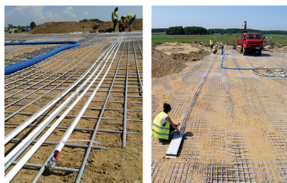
Fig. 7. Long base extensometers for measuring elongation of the steel grid
