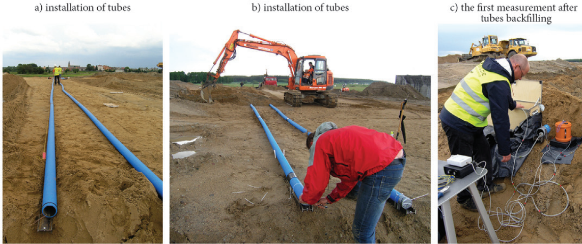
Fig. 8. Embankment settlement measurement by hydrostatic levelling
