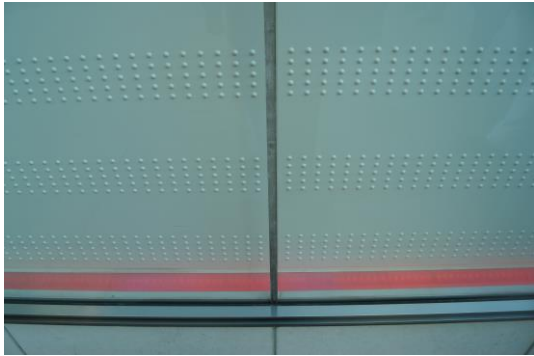
Fig. 15 Matsuya Ginza – detail of the curtain wall
