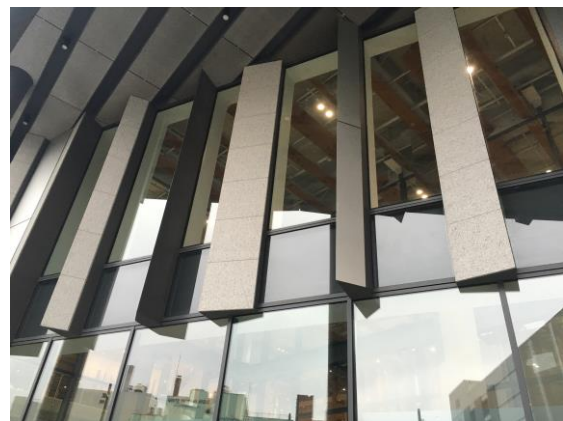
Fig. 34 Toyama Kirari – arrangement of panels
