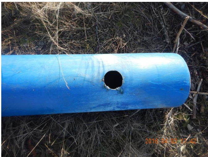
Fig. 12 Burned off whole that was initiated by the bullet and enlarged by oxidation
