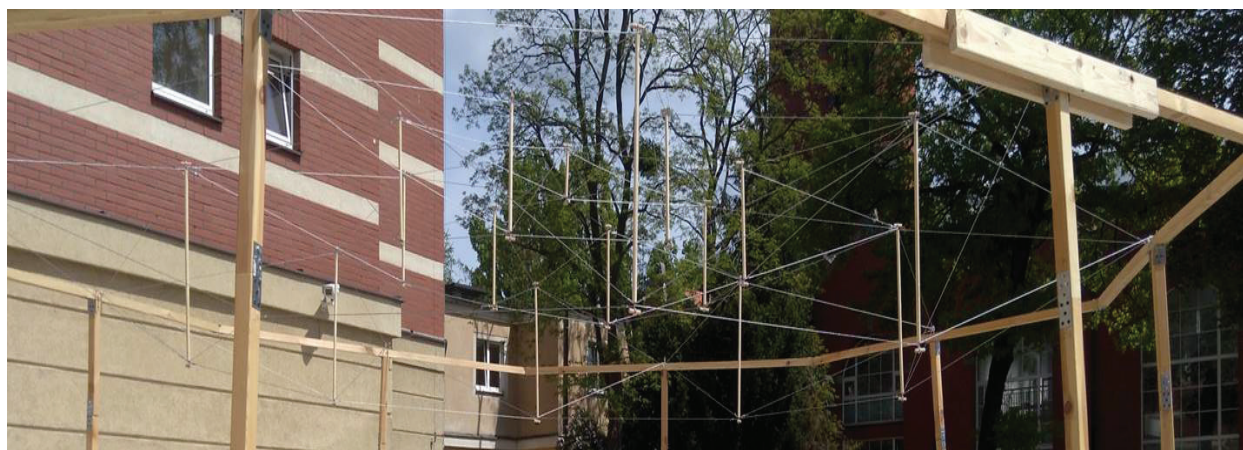
FIGURE 12. The erected real-life Fuller’s dome structure
