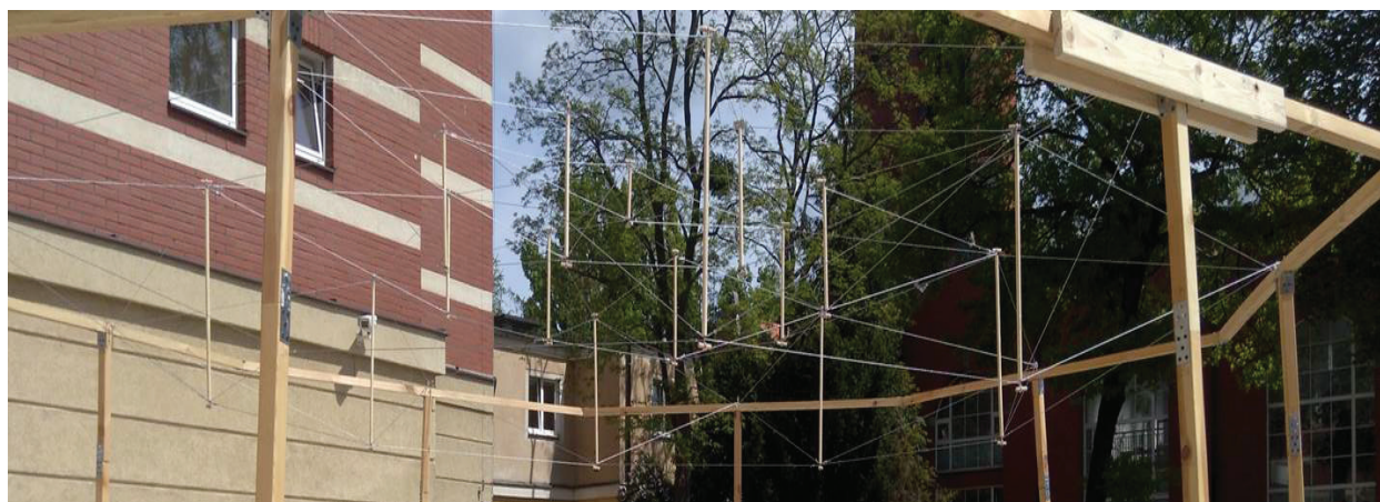
FIGURE 12. The erected real-life Fuller’s dome structure
