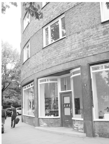
Photo 6. Multifamily building “Schichttorte” (Bahrenfelder Steindamm/Thomas Str.)
