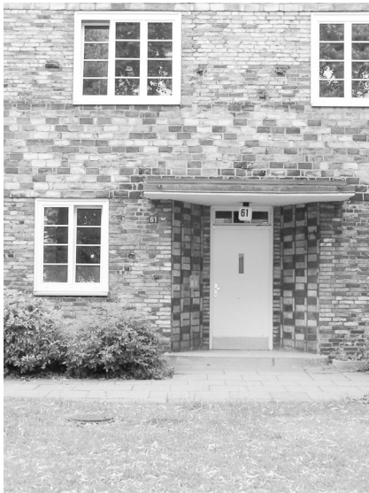
Photo 3. Articulation of the façade – Schützenstrasse multifamily house
