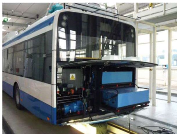
Fig. 3 Traction NiCd batteries (right) and DC converter (left)
