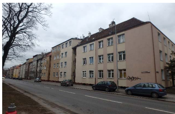
Figure 3. View of the building from the street [10]
