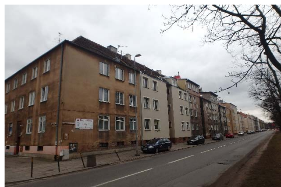
Figure 4. The view from the opposite side of the street [10]
