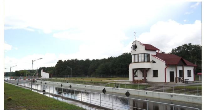
Fig 1. Water junctions no. 10 “Załużie” on the D-BC Source: Republican Unitary Maintenance and Construction Enterprise “Dnepro-Bug Waterway, Pinsk, Belarus
